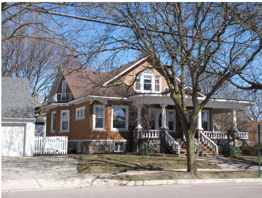
Main West 302_Looking Northeast
