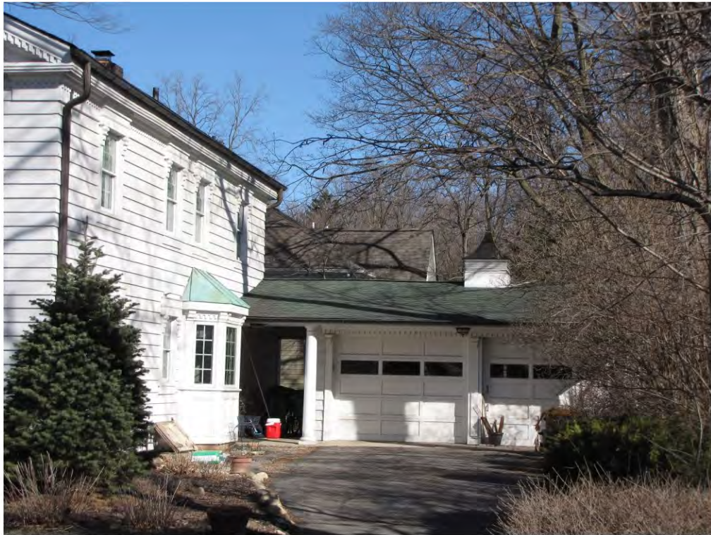
Randolph 204, Garage_Looking North
