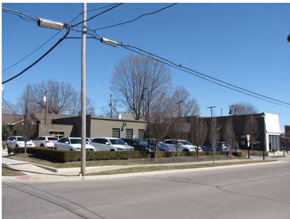
Main West 202_Looking Northeast
