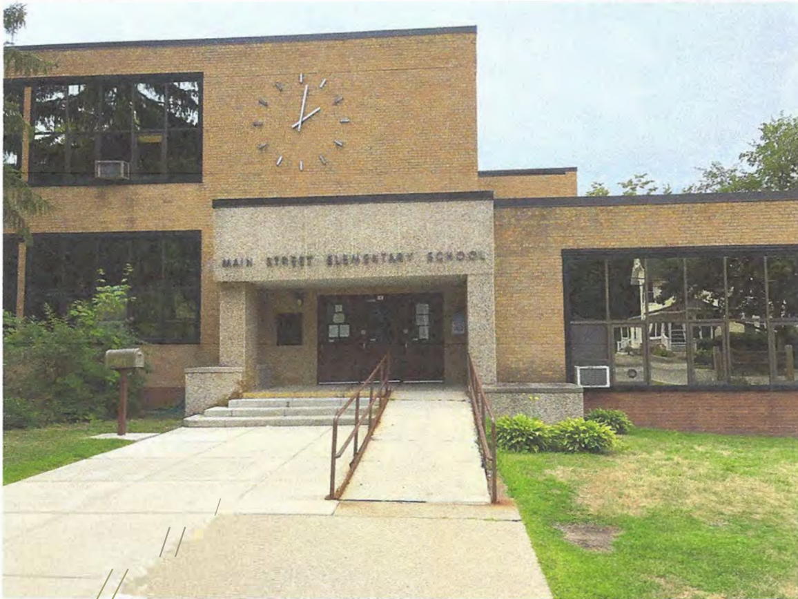
Current view of main entrance to building. Entrance was modified in 1970. The glass block windows above the doors were eliminated. Also, doors are now solid, whereas the architect originally designed them to be glass. Photo below documents date of remodeling.
