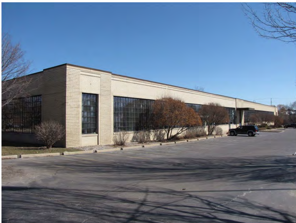
Main East 235 Looking Northeast
