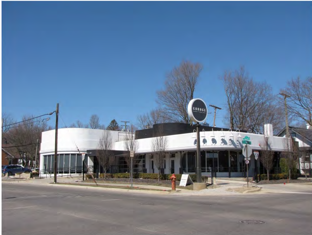
Main West 202_Looking Northwest
