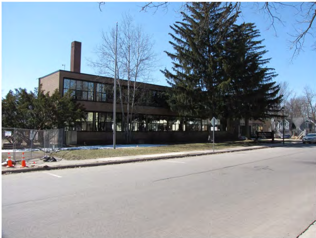
Main West 501_Looking Southwest
