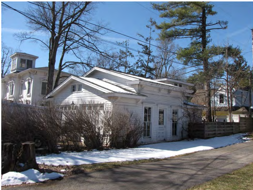
Dunlap West 404, Garage_Looking Southwest
