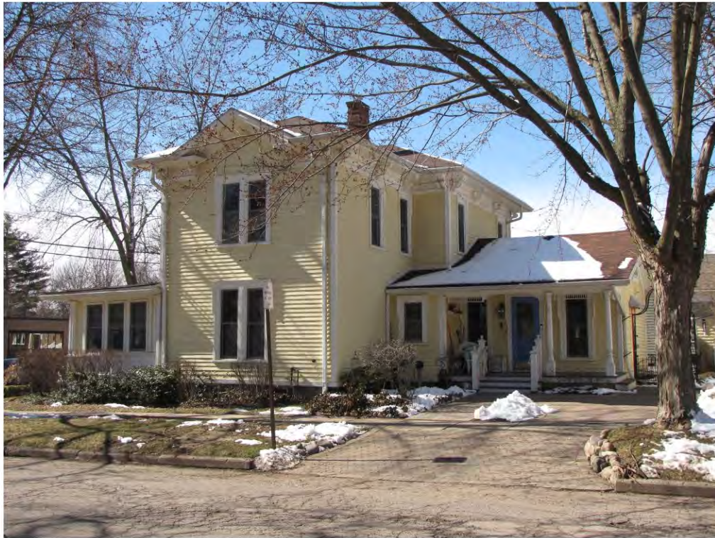
Main West 502_Looking Northeast
