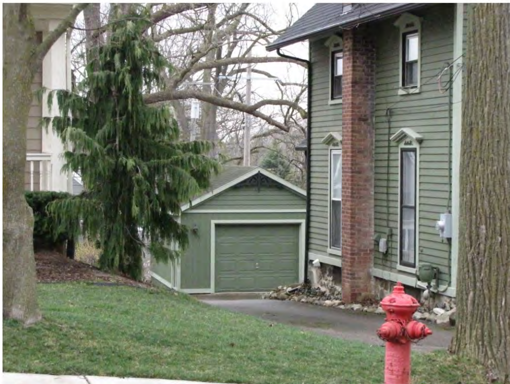
Rogers North 322, Garage_Looking East
