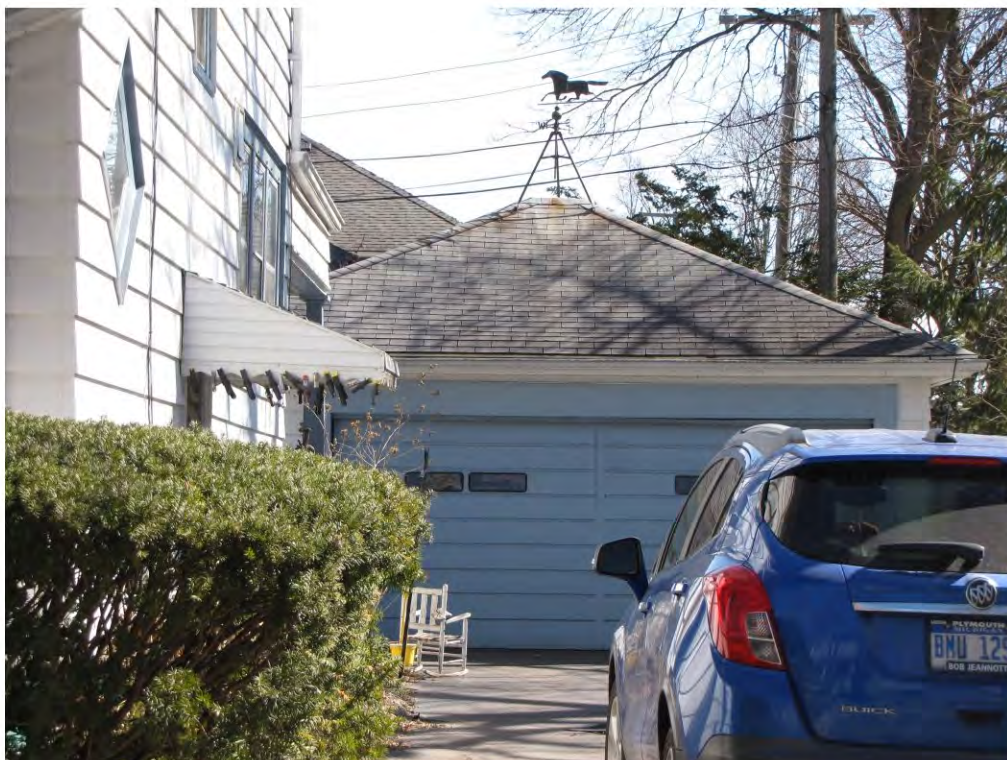
West 114, Garage_Looking East
