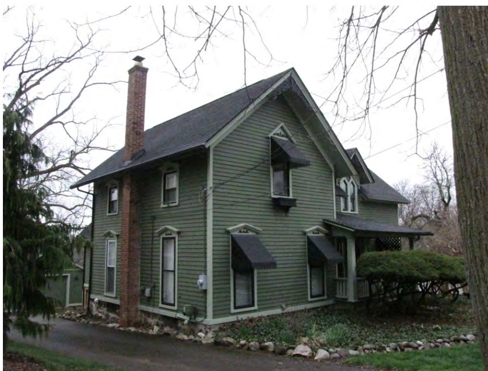
Rogers North 322_Looking Southeast
