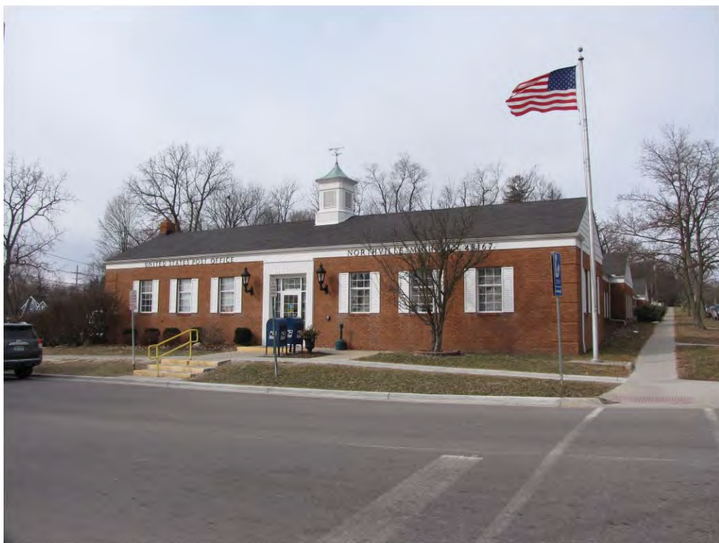
Wing South 200_Looking West
